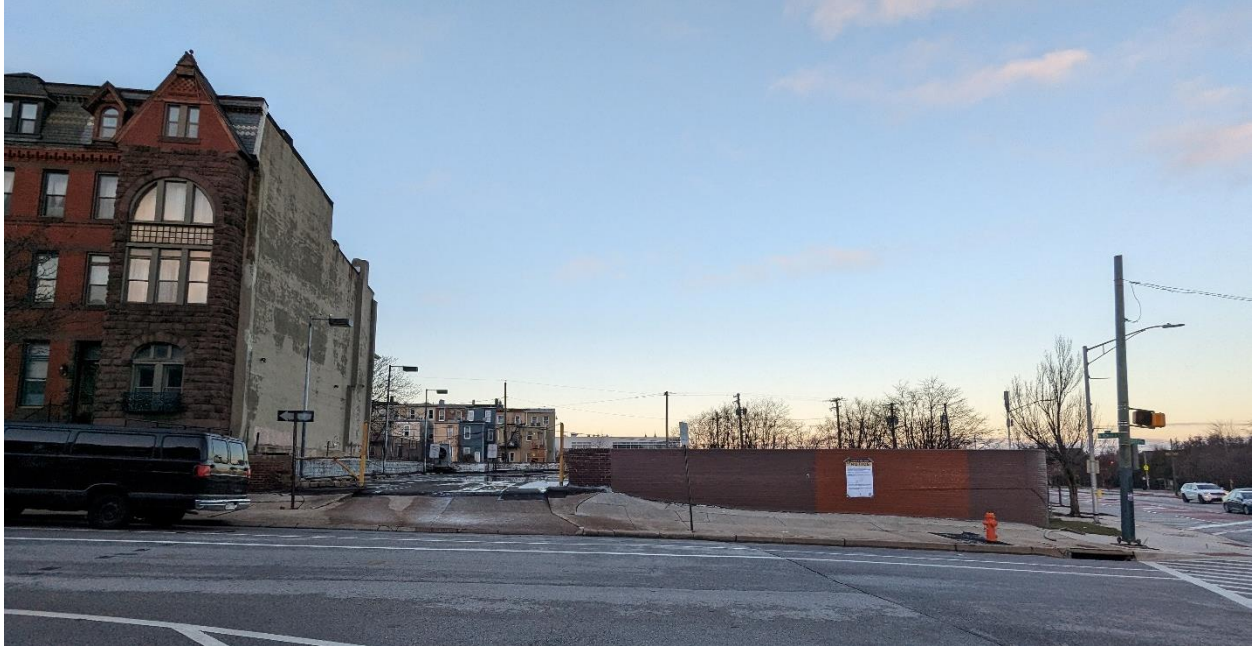
Fig. 21: View of the Eutaw Place elevation and rooftop parking deck of 920 W. North Avenue.
