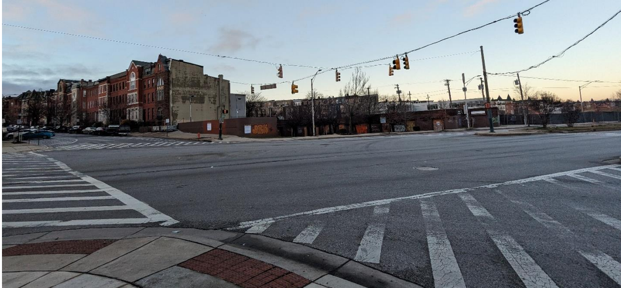
Fig. 14: View of 920 W. North Avenue from the southwest corner of W. North Avenue and Eutaw Place.
