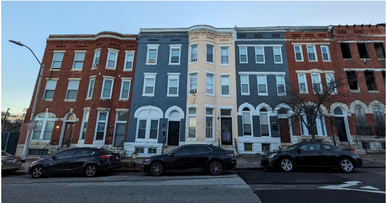
Fig. 28: Historic rowhomes on the side of the 2200 block of Linden Avenue that are immediately adjacent to the project site. These are located in the National Register Historic District of Reservoir Hill.
