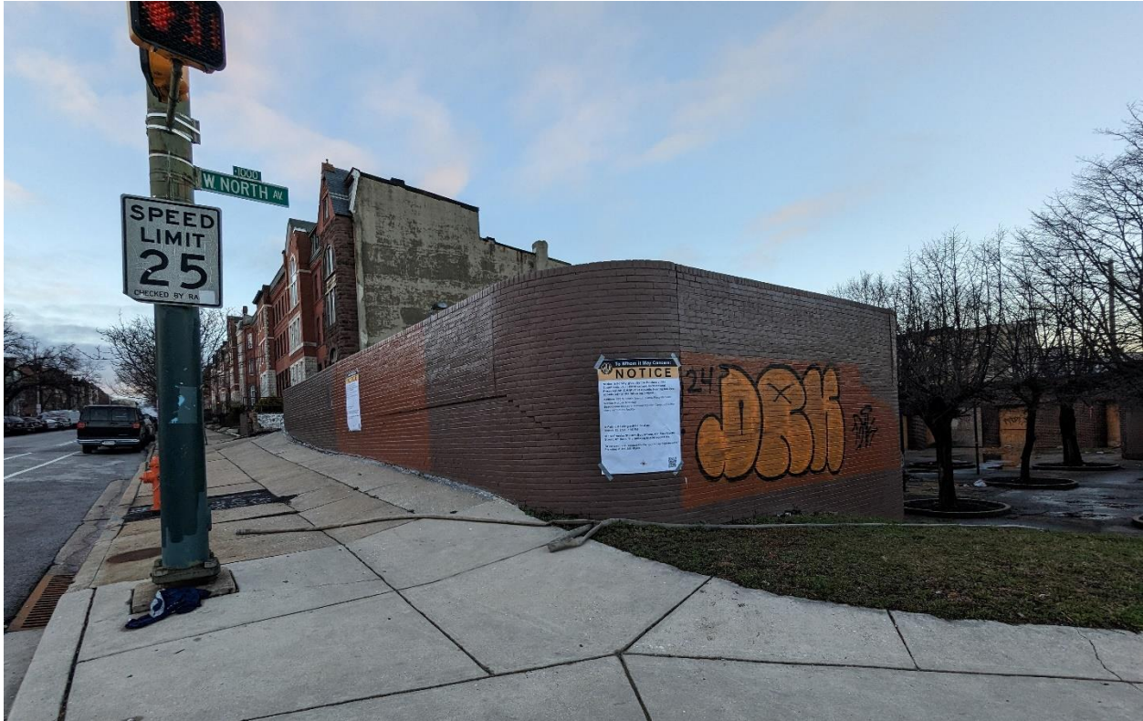
Fig. 17: Close-up view of 920 W. North Avenue along Eutaw Place, as viewed from W. North Avenue.
